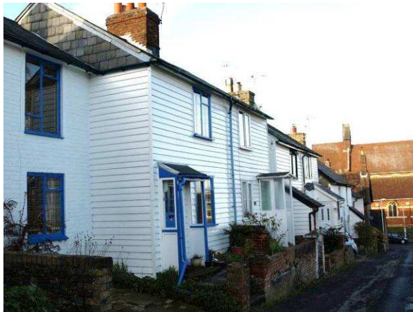
West side of Prospect Road
