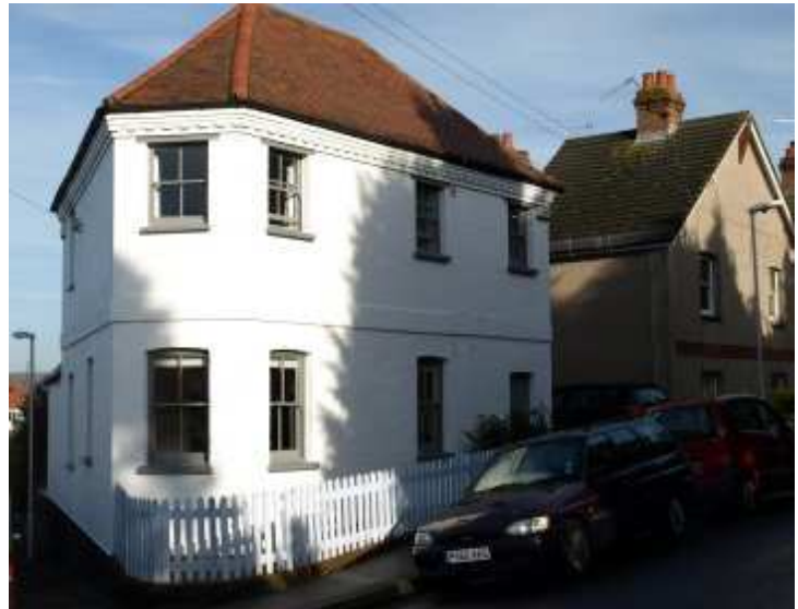
43 Hartslands Road – former corner shop with picket fencing
