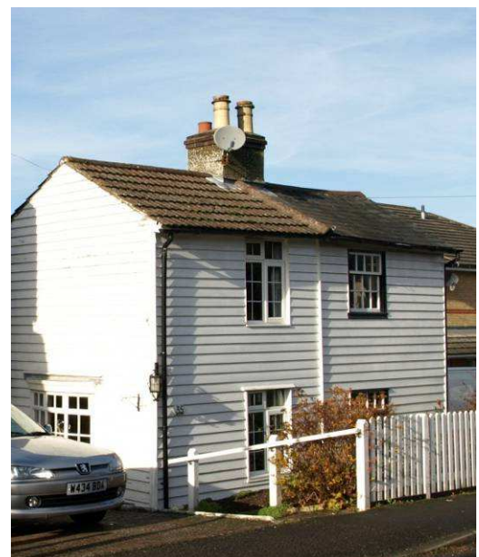
35 and 37 Hartslands Road – white weather boarded possibly former farm cottages with white picket fencing
