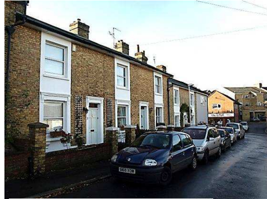
South side of Cedar Terrace Road
